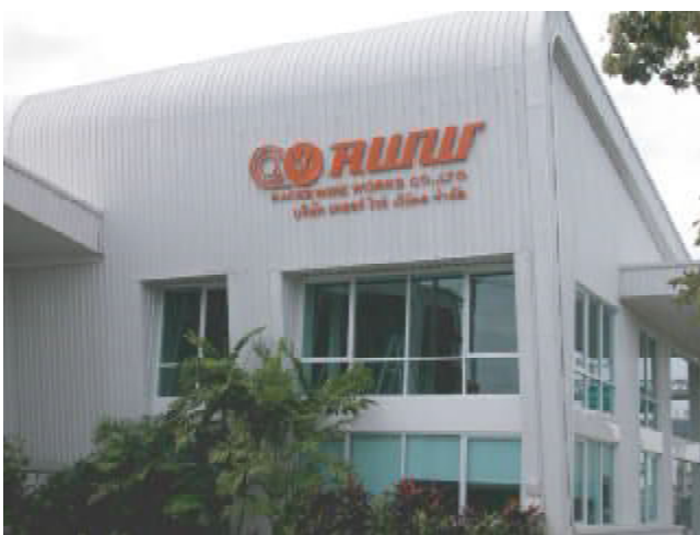
Racer Wires Work co.Ltd.
